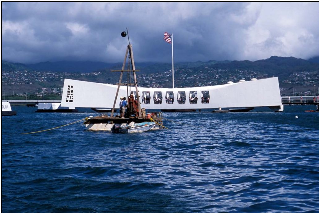
Figure 10.6. A small anchored barge was used to advance the borehole. The deck and railings of USS Arizona are completely submerged in 2003, with the vessel tilting several degrees to the southeast (USGS Photo).
